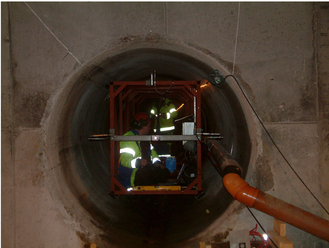
Figure 2-1 Control measurements of horizontal deposition hole (KBS-3H).
