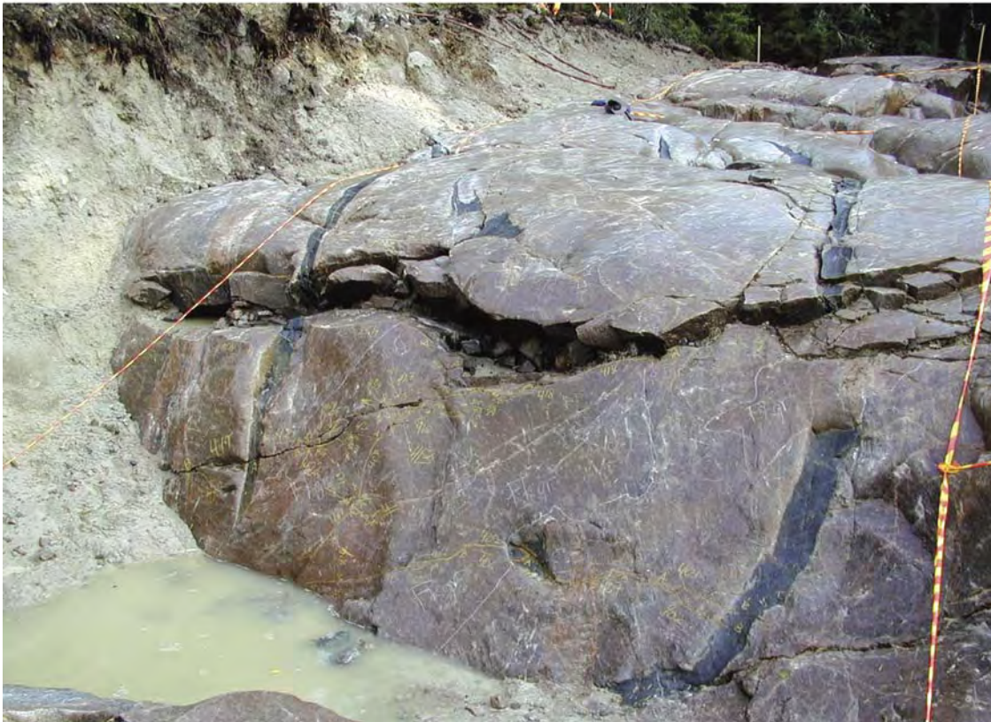
Figure 4-4. Two of the predominant, gently dipping fractures containing sediments, both viewed from northwest. The lower photo also illustrates the uplift of the superficial rock overlying these fractures.
