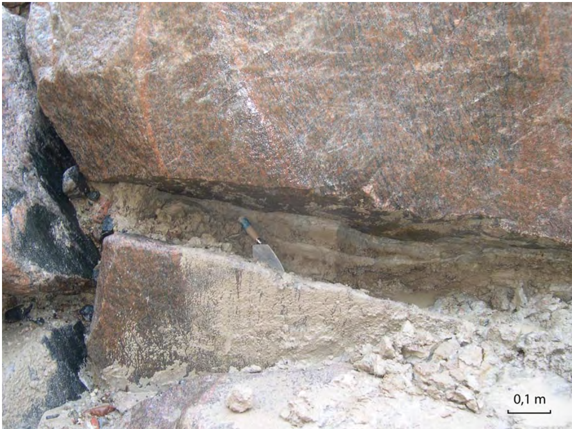
Figure 1-4. Example of a gently dipping fracture, more than 10 cm wide and filled with sedimented soil material.
