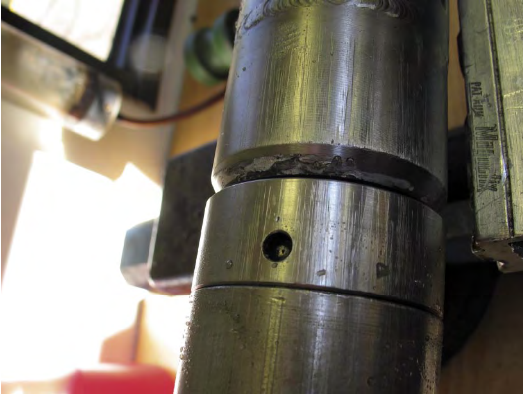
Figure 2-9. Details with crevice corrosion inside the chemical analysing equipment.
