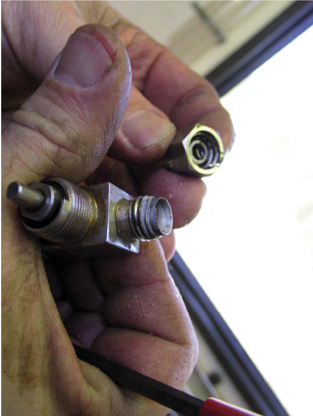
Figure 2-4. Corroded thread and nut on a valve inside the chemical analysing equipment.
