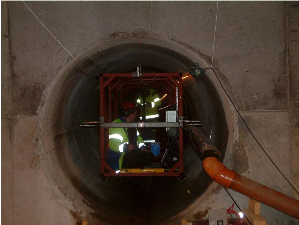
Figure 2-1 Control measurements of horizontal deposition hole (KBS-3H).
