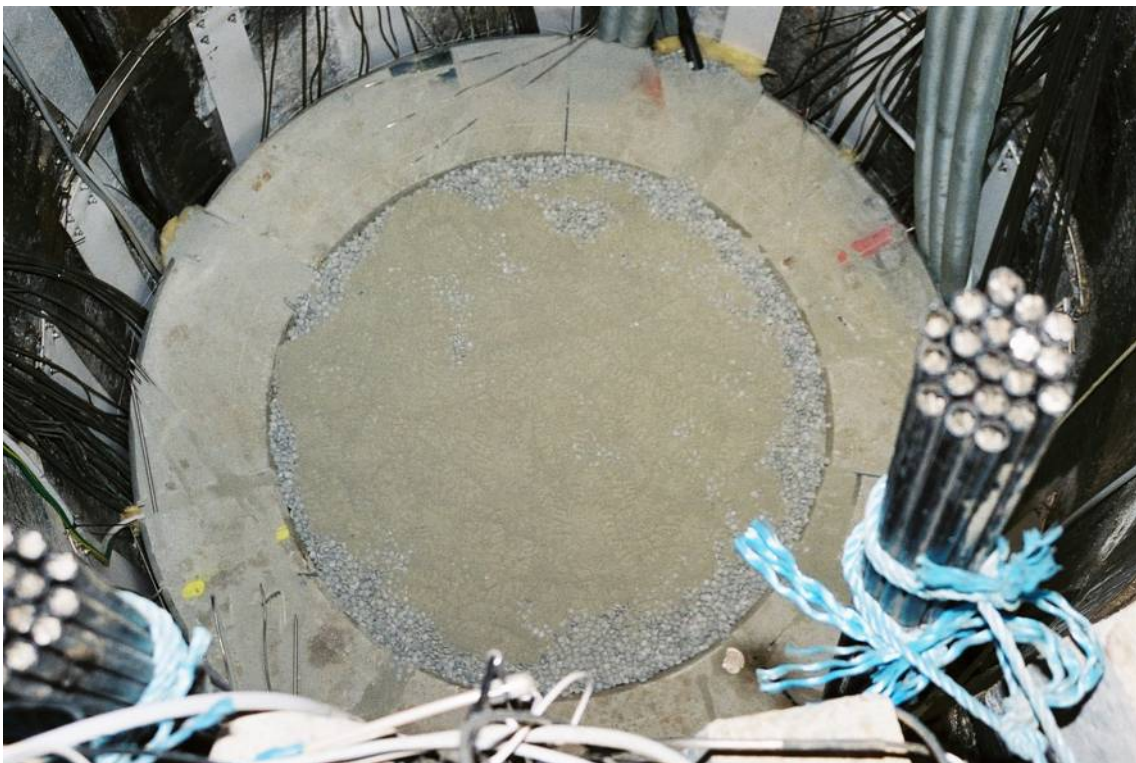
Figure 5.3-10. Pictures taken after emplacement of the bentonite bricks on top of the canister (upper) and after supplementary filling with pellets and powder (lower).
