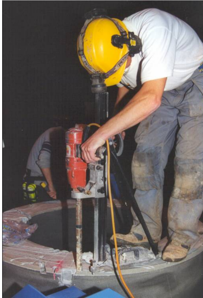
Figure 5.3-6. Preparation of bentonite ring R10.
