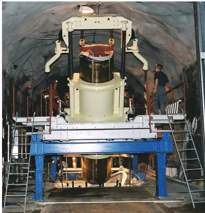
Figure 5.4-1. Raising of canister to an upright position
