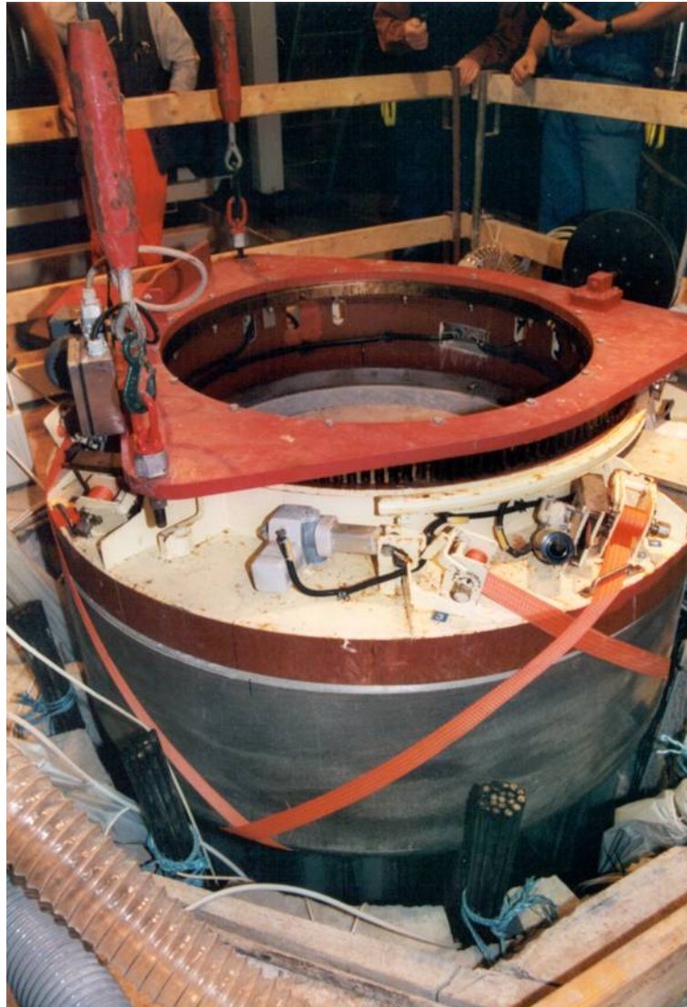
Figure 5.3-7. Placement of a bentonite ring.
