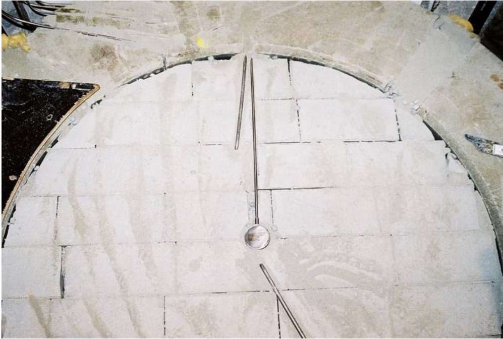
Figure 5.6-1. Picture taken after placement of the bentonite bricks on top of the canister and installation of three instruments.
