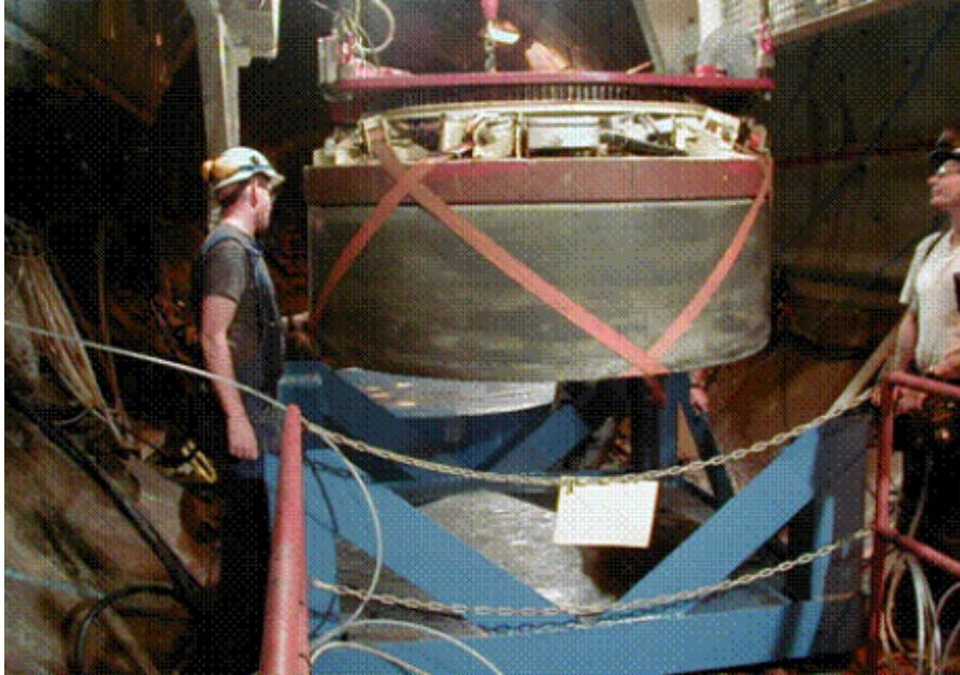
Figure 5-22. Application of a 2 Mg precompacted buffer block of MX-80 bentonite in a KBS-3V type waste emplacement hole [5-16].
