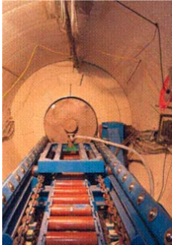
Figure 5-20. Appearance of buffer blocks placed in the Febex test drift at Grimsel [5-15].
