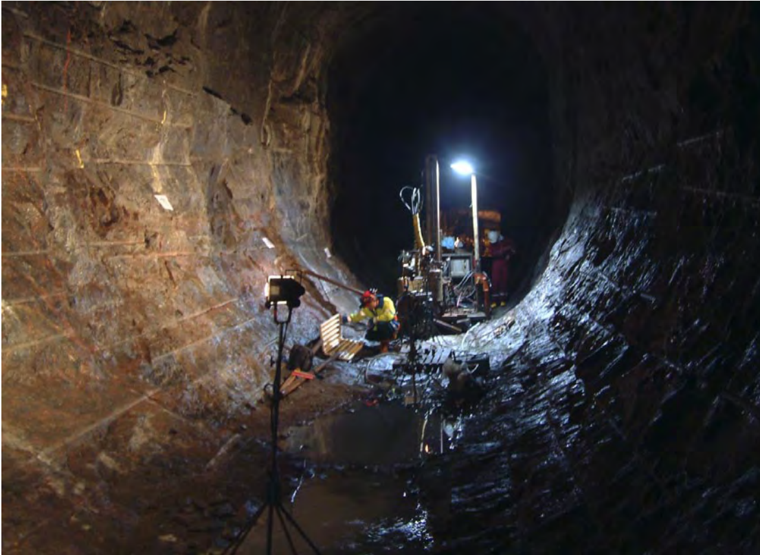
Figure 3-1. The experimental TASQ drift shortly after the excavation.
