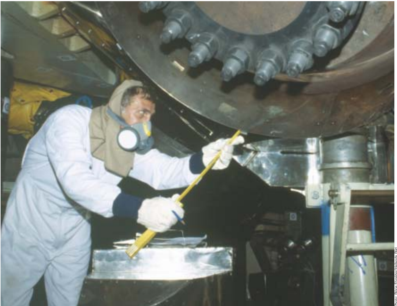
All surfaces that have been in contact with the water in the reactor are more or less contaminated with radioactivity.
