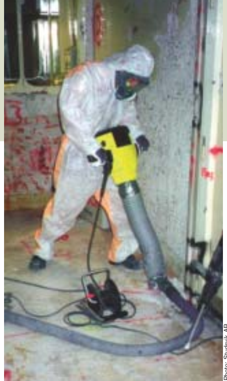
Contaminated areas are drilled away and disposed of.
