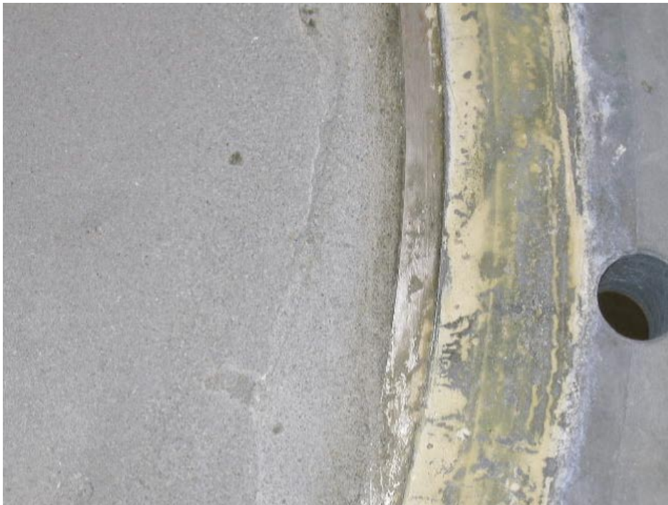
Figure BB3-3. Picture showing the sealed slot.
