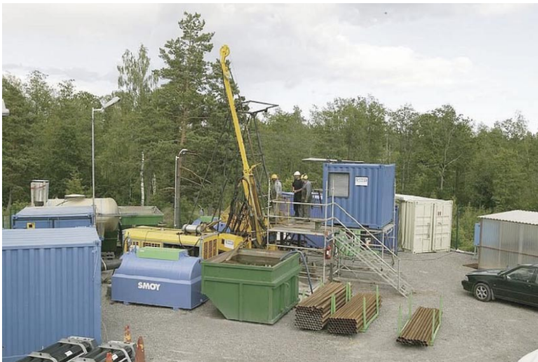
Figure 4-1. The KLX03 drill site.
